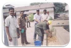
Building with bricks made out of waste black sand
